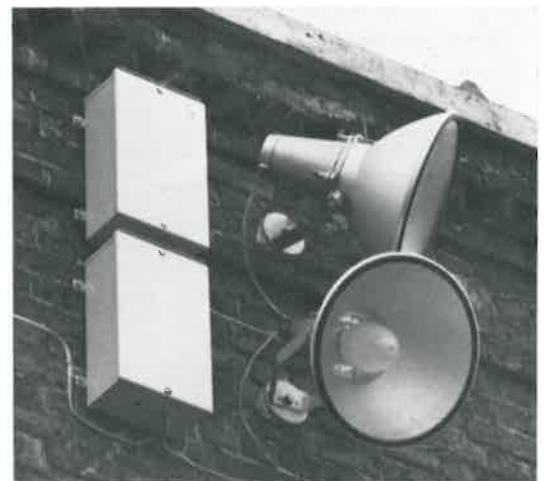
The plan above shows the location of Atlas M 25 projectors on buildings surrounding the Town Hall. Two, each containing a 400W SON lamp, are seen with their control-gear boxes.
