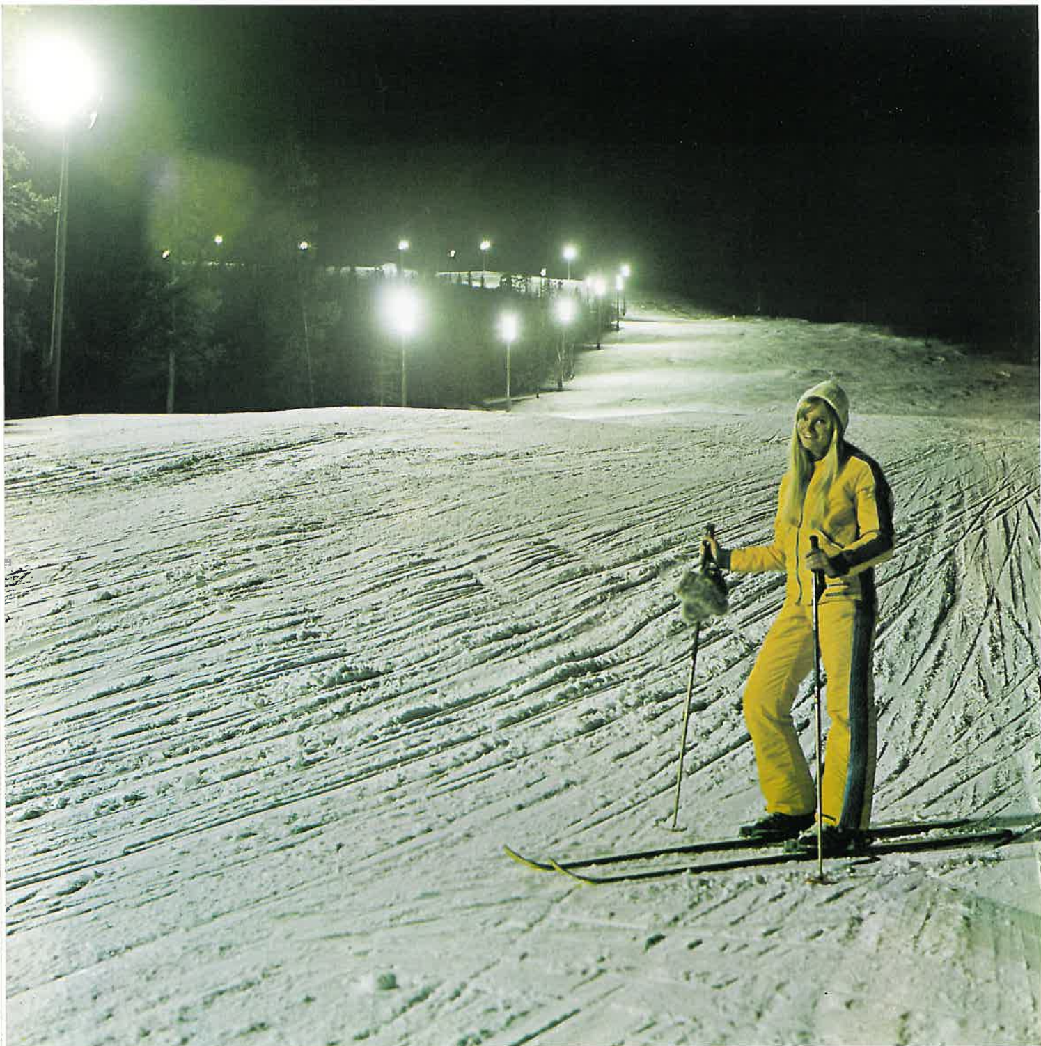
The slalom track at Dundret in Sweden, lit by Kolorlux lamps in M 25 fittings. Each of the 24 columns carries four narrow-beam and two dispersive fittings.
