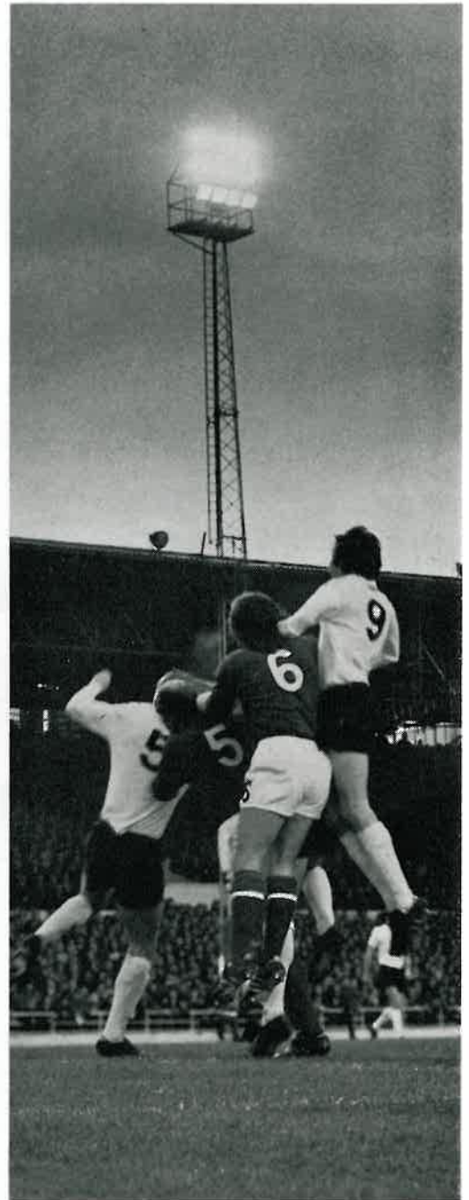
Each of the eight 30m towers at Luton Town carries twelve 1600W MBIL/H lamps in Atlas floodlight fittings.
